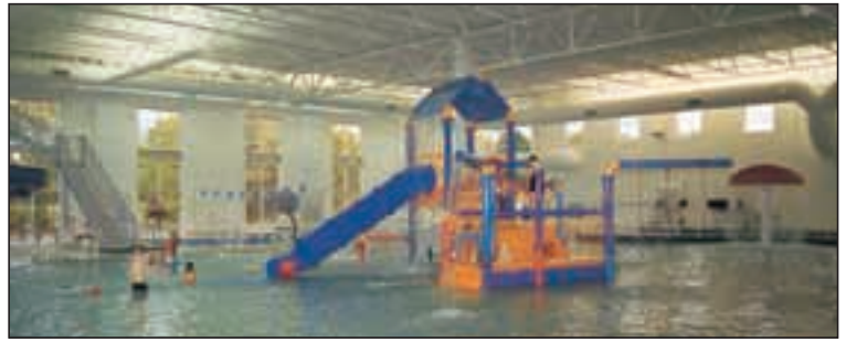
The 17,000 sq. ft. water park at Motion Fitness features three pools, a whirlpool and fun for the kids. Attractive white light is provided by 80 ft. lengths of 400 watt metal halide lamps.
