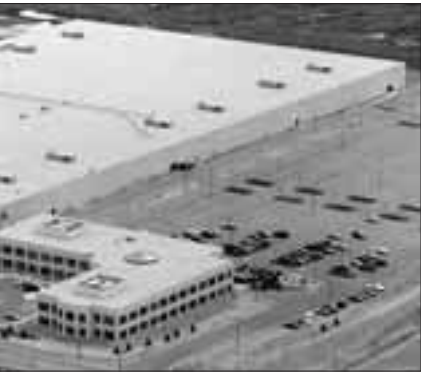
21.6 billion global giant, relocated its es to this 600,000 sq. ft. plant in ovated the plant which was built by
