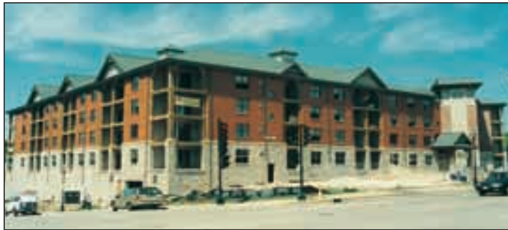
The Landing, a luxury corporate and short-term apartment complex, is under construction in downtown Waukesha. Steve Kassens, construction manager for builder/developer Harmony Homes, said, "We're using Roman for everything they do: electrical construction, telephone, data cabling, and the infrastructure for our Local Area Network."
